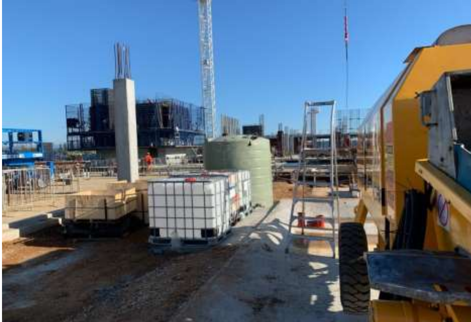
Photo 4 Bunded area for Concreting Works
