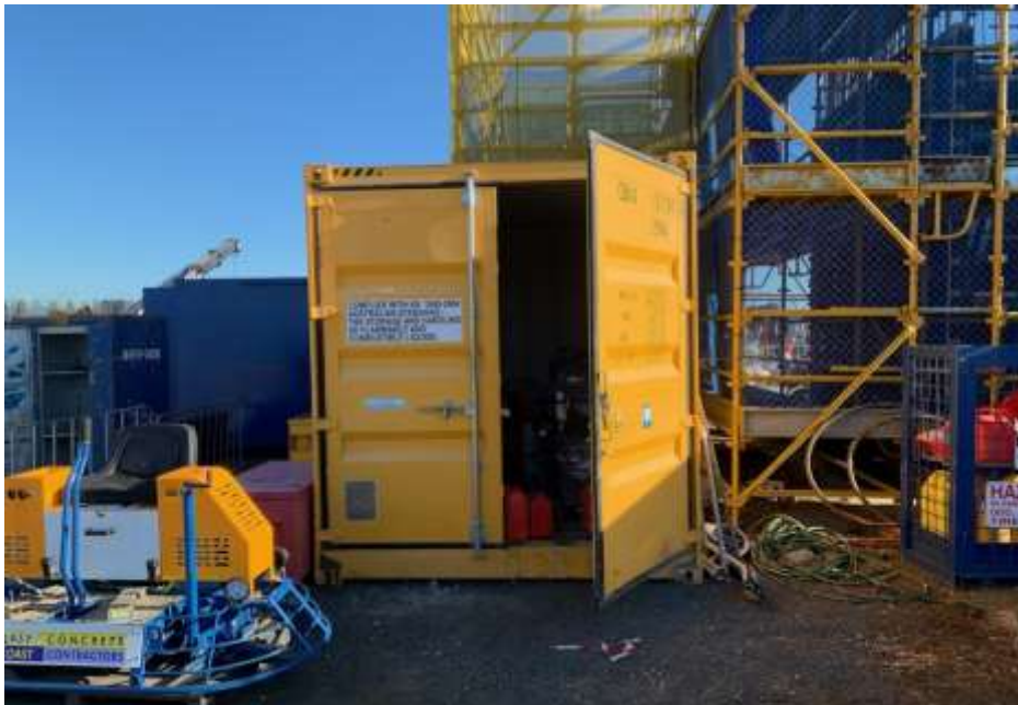
Photo 5 – Chemical Storage Container – bunded and ventilated
