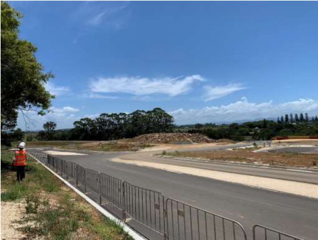
Photo 3 Stockpile Site and Sealed Access Road
