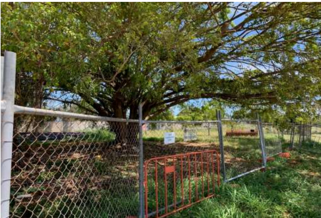
Photo 4 Tree Protection and Signage
