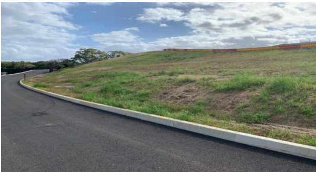
Photo 2: Stabilised Site Batter providing protection against Erosion and Sealed Access Road.
