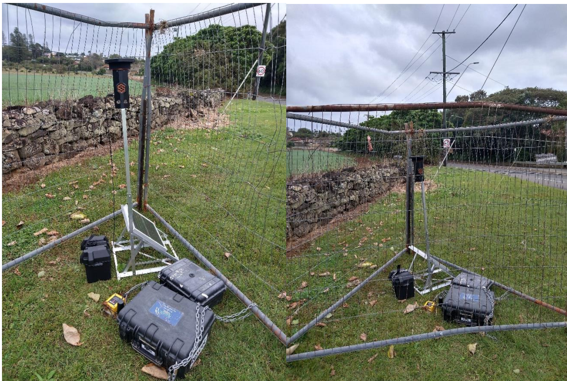
Figure 3-1 Noise, dust and vibration monitor installation locations
