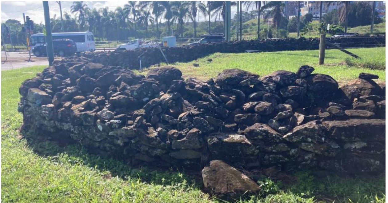
Figure 6-2 Dry stonewall on the south-eastern corner of the intersection. This wall will be impacted by the works, however, was determined not to be locally significant and will be rebuilt.
