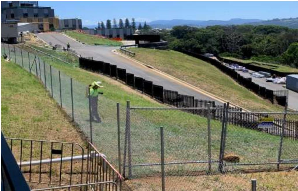
Photo 2 Internal roadworks completed with improved batter stabilisation (weed control being undertaken)
