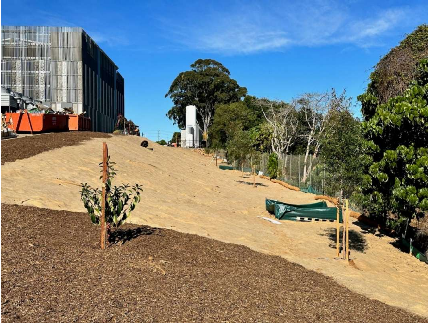
Photo 7: Landscaping works and sediment control measures
