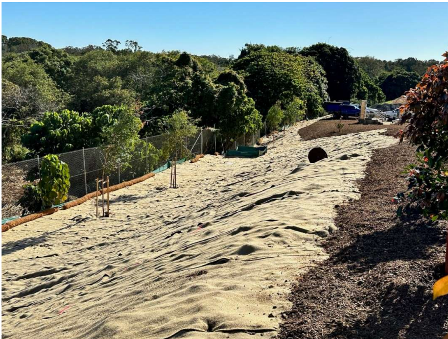
Photo 8: Landscaping works and sediment control measures
