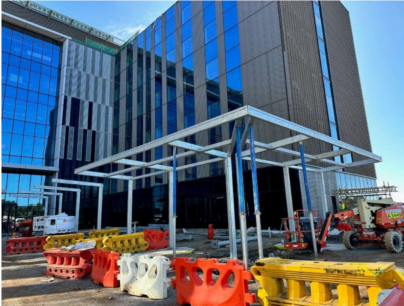
Photo 1: Construction of main hospital building nearing completion
