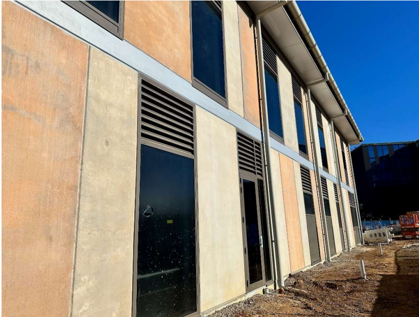
Photo 3: Construction of the Health Hub external facade
