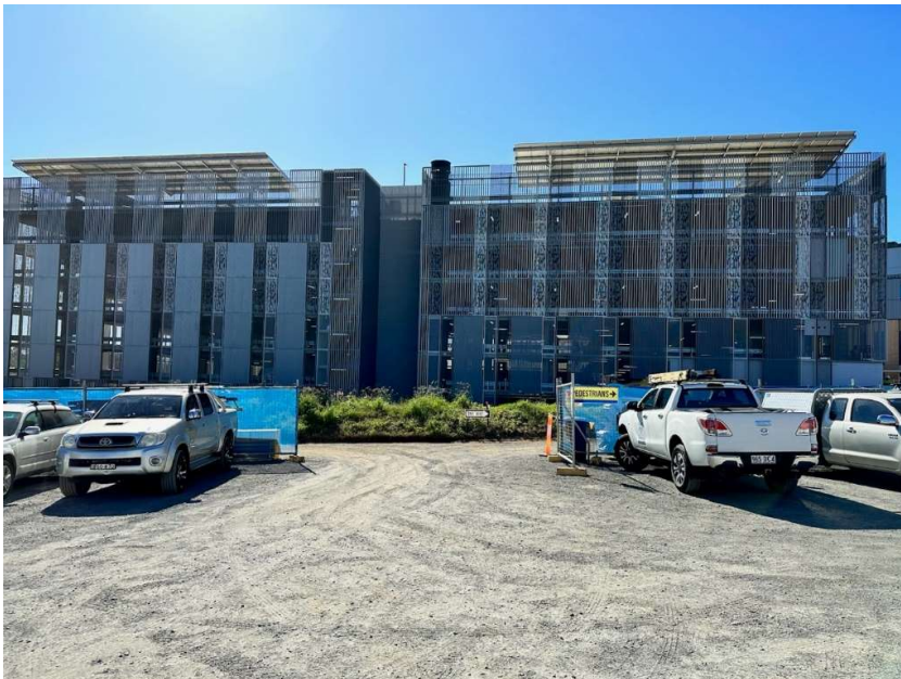
Photo 2: Construction of the carpark nearing completion
