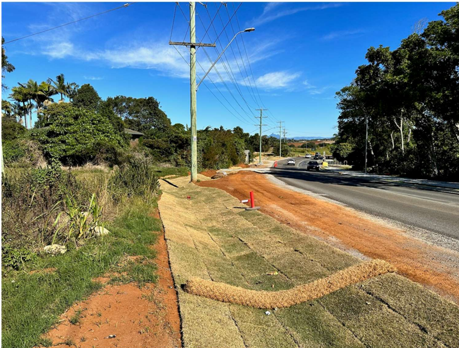
Photo 12: Permanent swale drain
