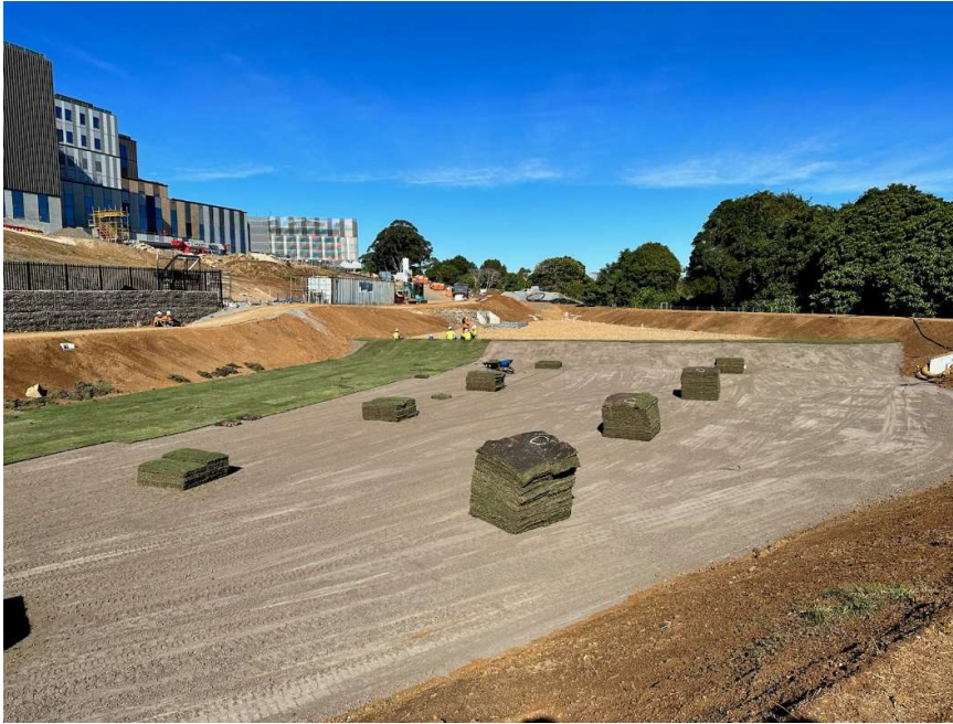
Photo 5: Construction of bioretention basin (underway)
