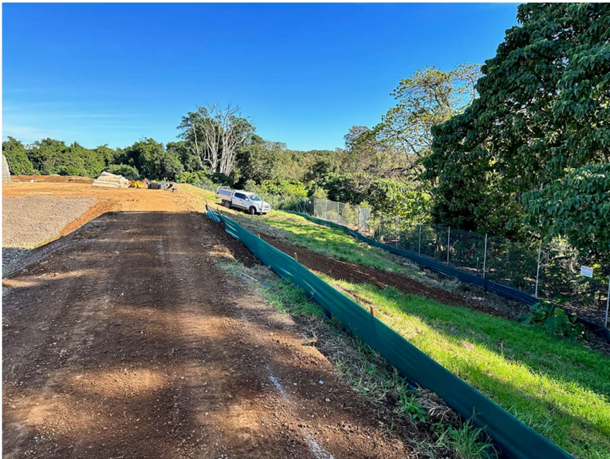
Photo 6: Erosion and sediment control and batter revegetation
