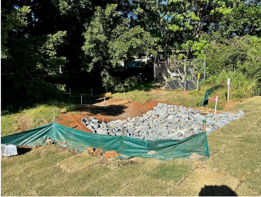
Photo 11: Permanent drainage work, Cudgen Road
