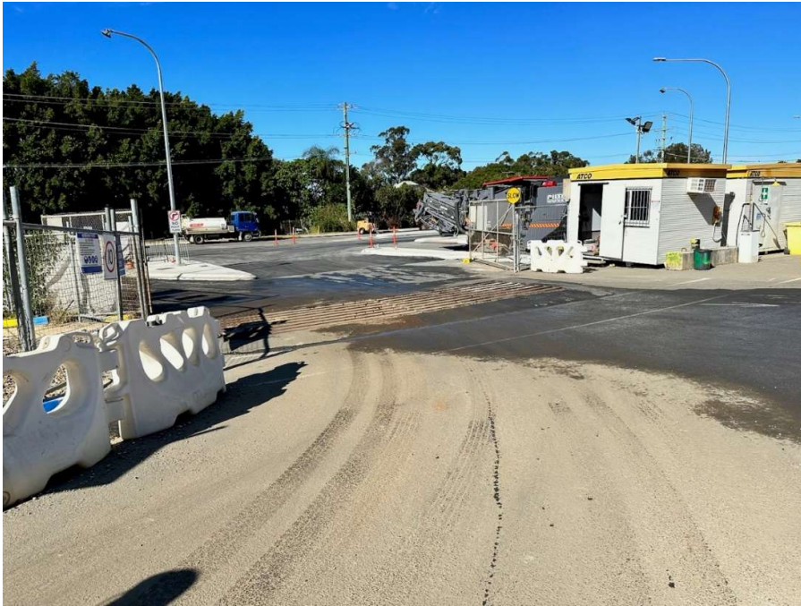
Photo 9: Stabilised site access and vehicle entry/egress point – ADCO site
