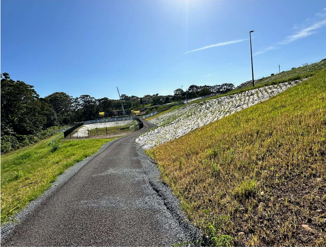
Photo 2: Stabilised and completed batter with permanent drainage basin installed
