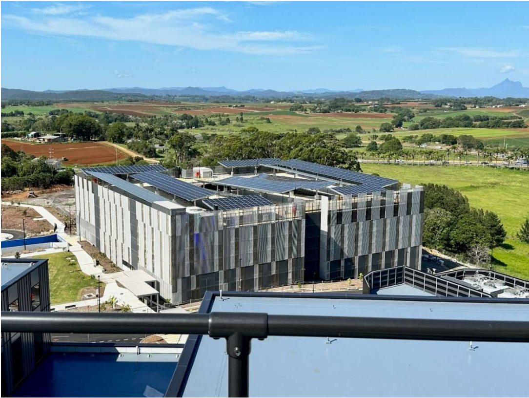
Photo 3: Completed carpark with solar panel roofing
