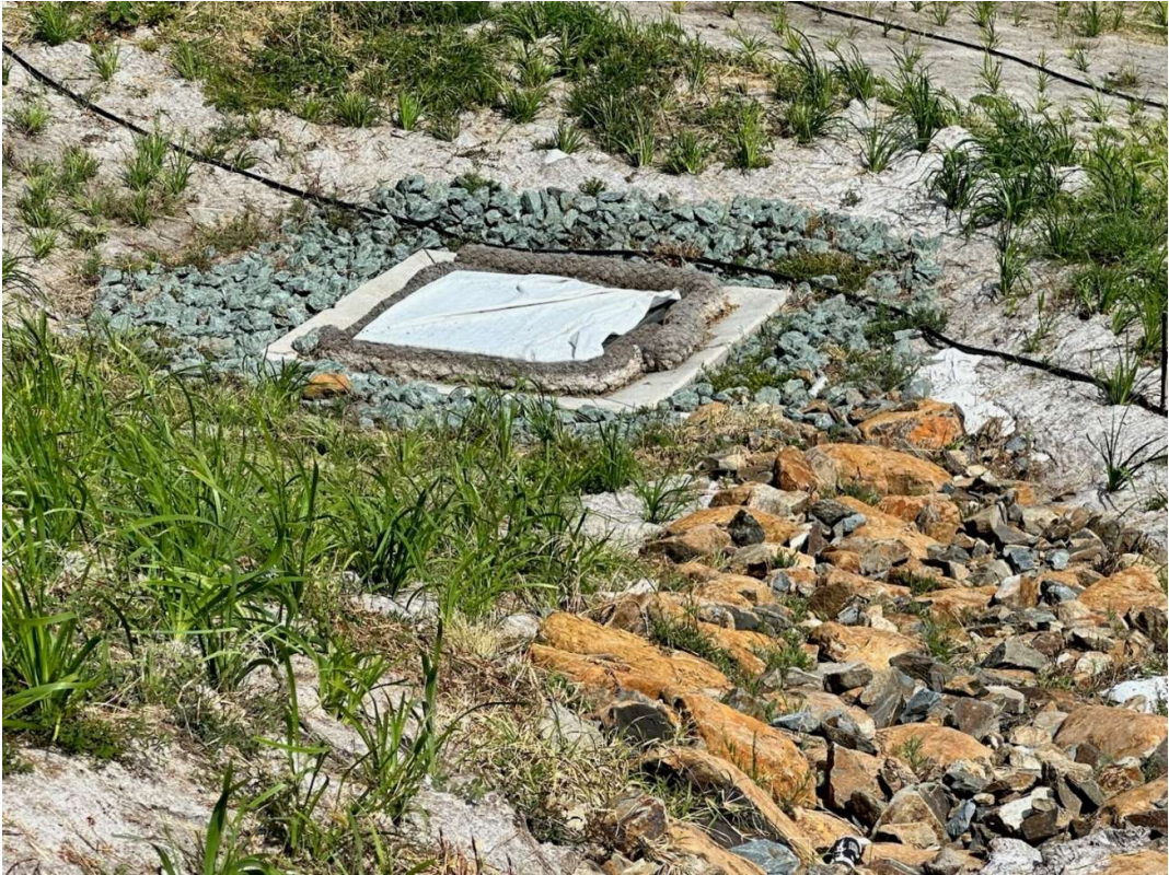
Photo 4: Permanent drainage and pit protection
