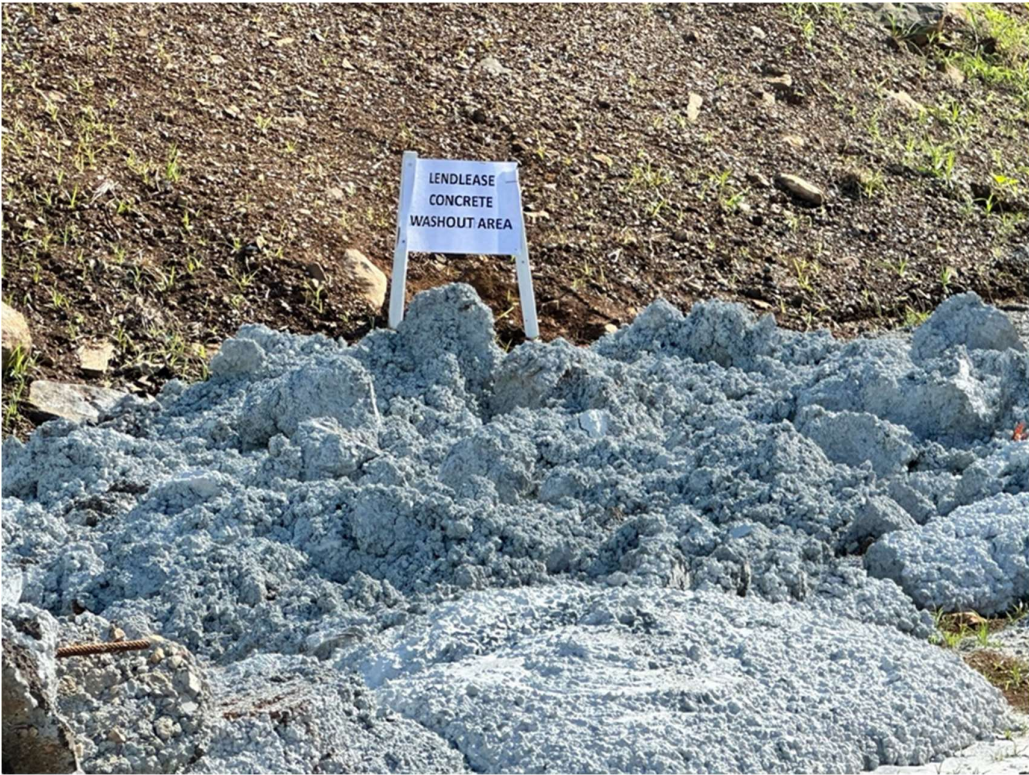
Photo 13: Concrete washout pit
