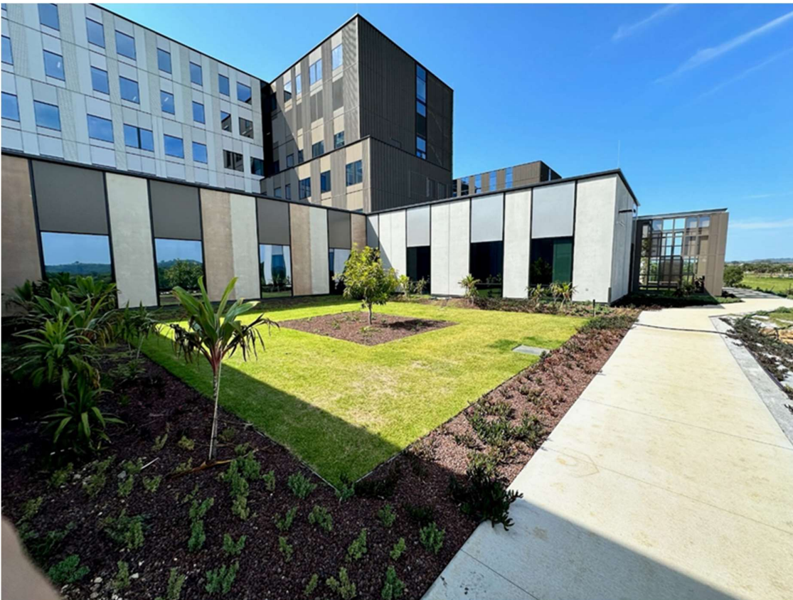
Photo 1: Main Hospital Completed
