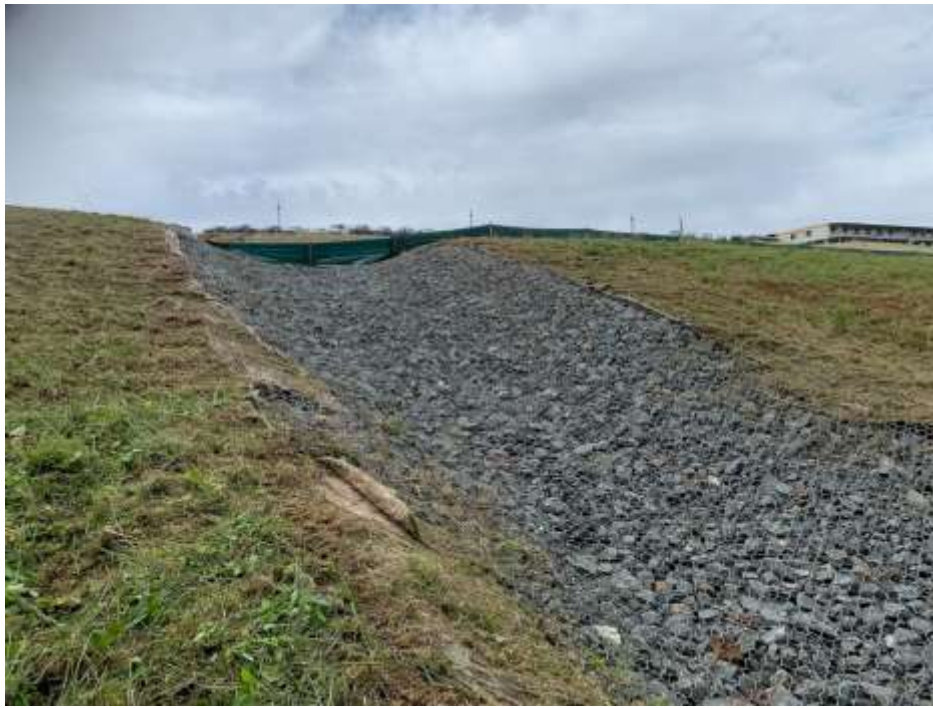
Photo B1.5: Permanent Scour Protection – Sediment Basin
