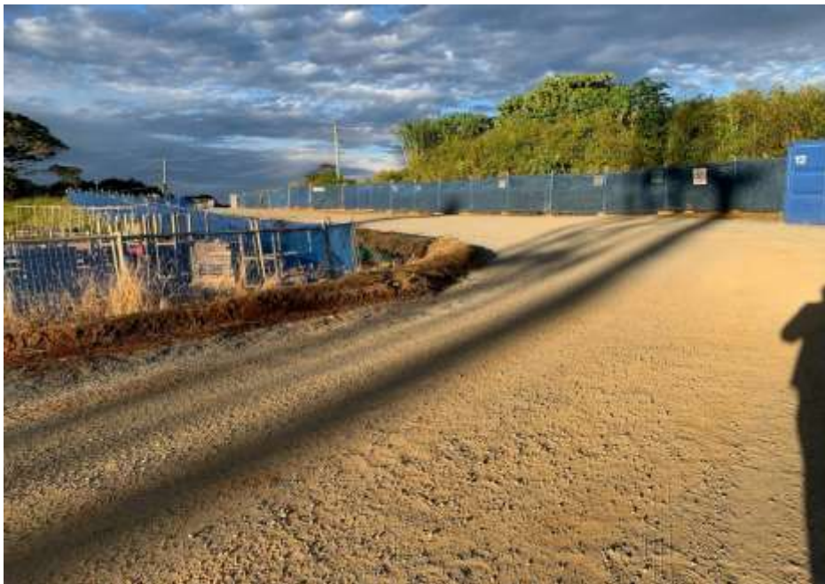
Photo B 2.2: Site Access Road
