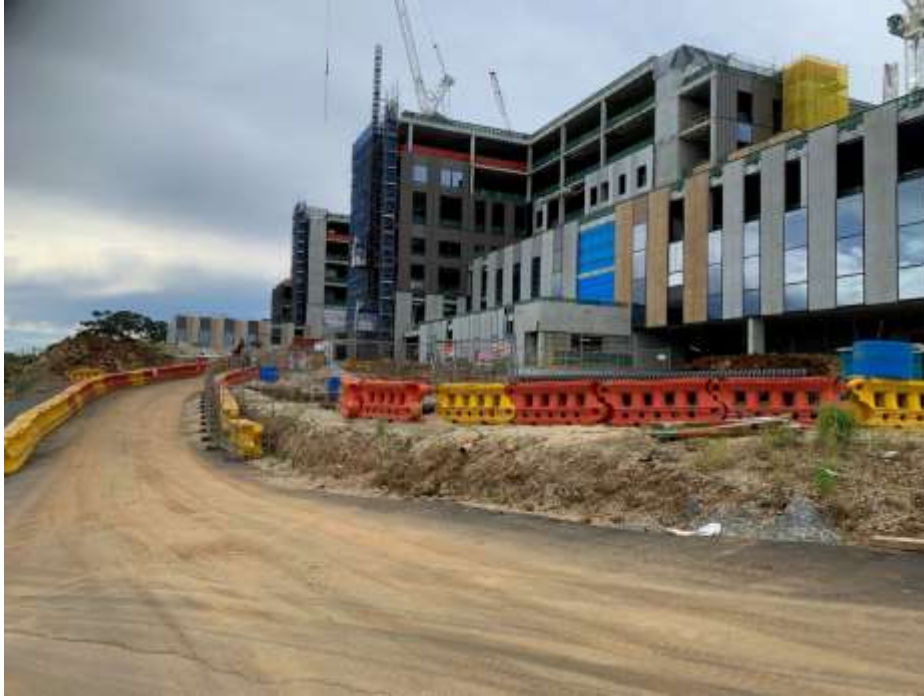
Photo B1:1 Construction of main hospital building with façade progressing
