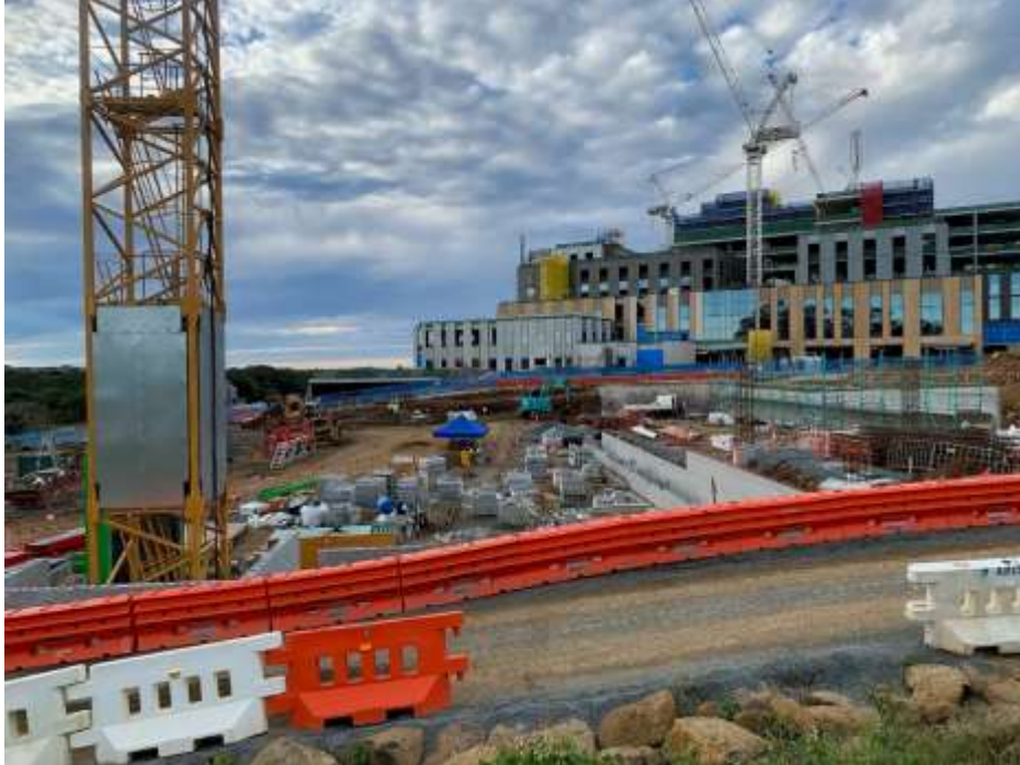
Photo B 2.1: Carpark Construction Site
