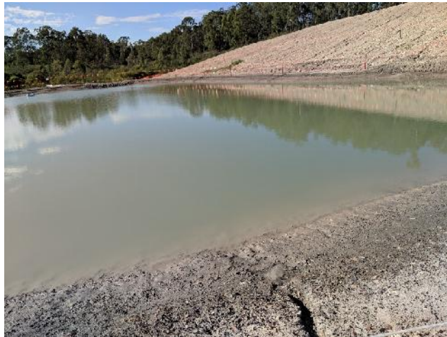
Figure 1: Sediment basin to manage rainwater retention on site
