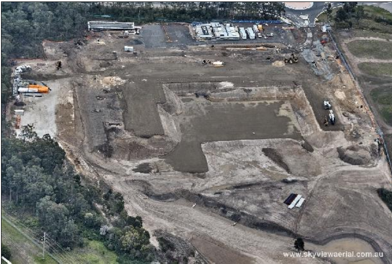
Figure 5: Aerial Shot of the general site and construction activity.
