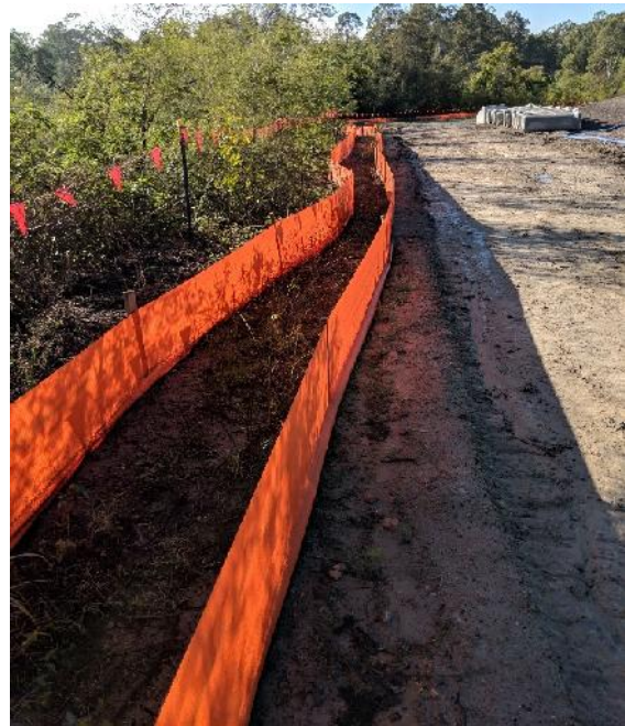
Figure 2: Sediment control in place
