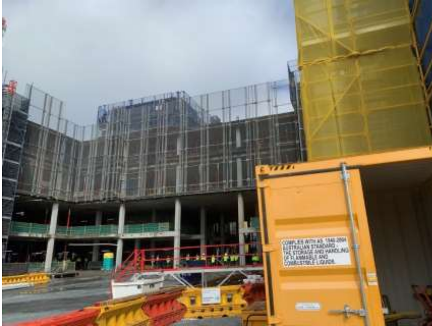
Photo 1: Building structure and scaffolding
