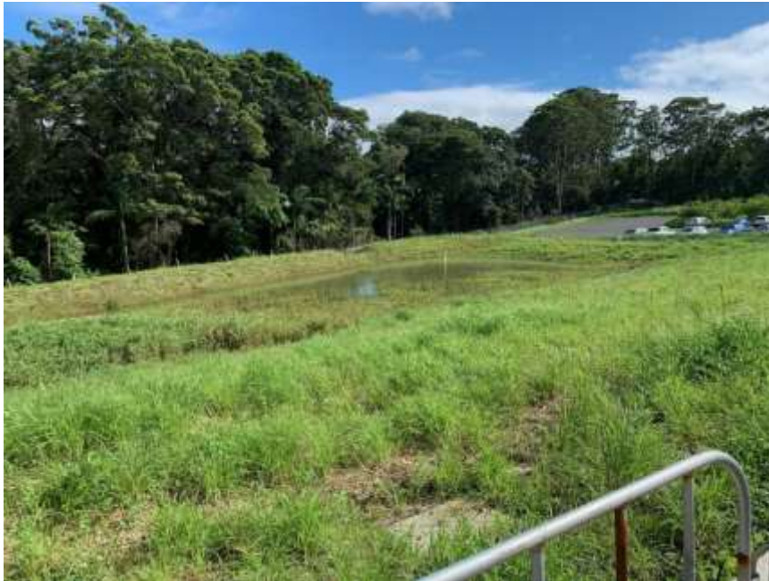
Photo 6 – Sediment Basin in operation
