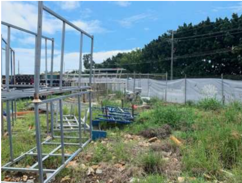
Photo 2: Environmental Monitoring Station
